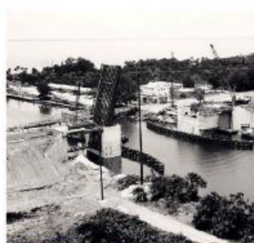
Construction on Haulover Canal in the new area. This is the same foot print we use today, including a draw bridge to allow for larger vessels. Photo courtesy of NASA Kennedy Space Center Archives
