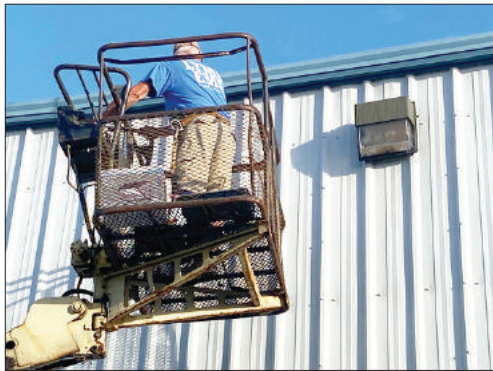
Roger Tonovitz replacing lights
