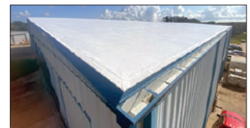
New roof South side
