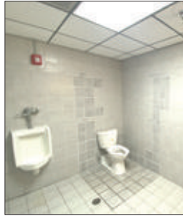
Bathroom Renovation before partition
