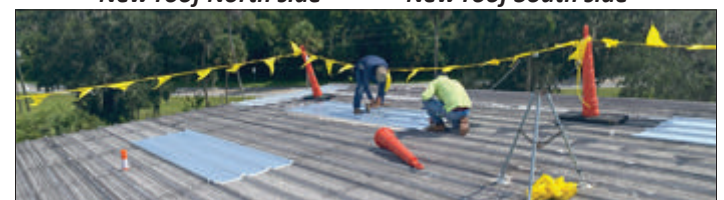
Covering skylights on roof before TPO installation
