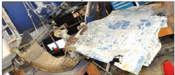
Horizontal Stabilizer • before
