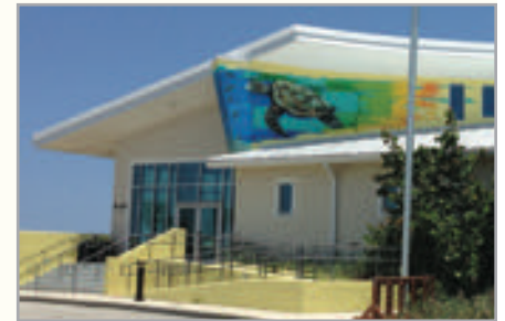
Barrier Island Center
