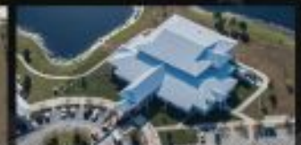
WICKHAM PARK COMMUNITY CENTER
