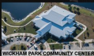
WICKHAM PARK COMMUNITY CENTER
