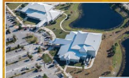
Wickham Park Community Center
