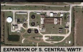
EXPANSION OF S. CENTRAL WWTF
