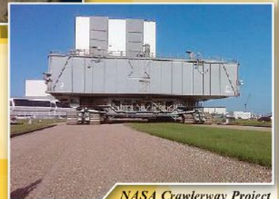
NASA Crawlerway Project
