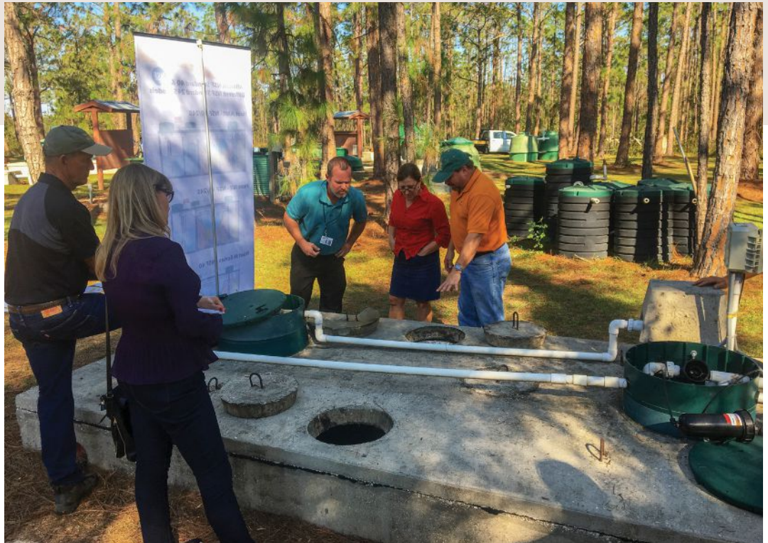
County staff and members of the Citizens' Oversight Committee visiting the Florida Onsite Wastewater Association Training Center in Lake Alfred to see dozens of advanced septic system technologies in action, meet with the design engineers, and discuss innovative opportunities for sewage treatment.
