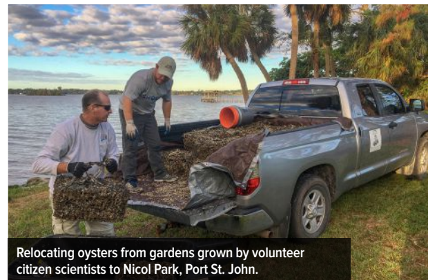
Staging bags of oyster shell for construction of an oyster reef breakwater at Geiger Park, Melbourne.
