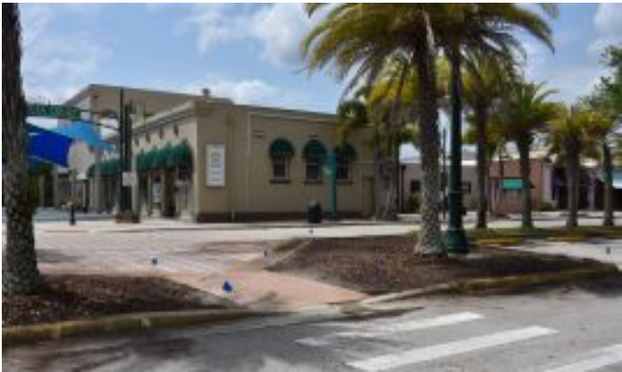
Landscaping improvements are being done at the Commons Parking Lot. Landscape improvements on Washington Avenue and Hopkins Avenue between South Street and Grace Street are proposed to take place this summer.
