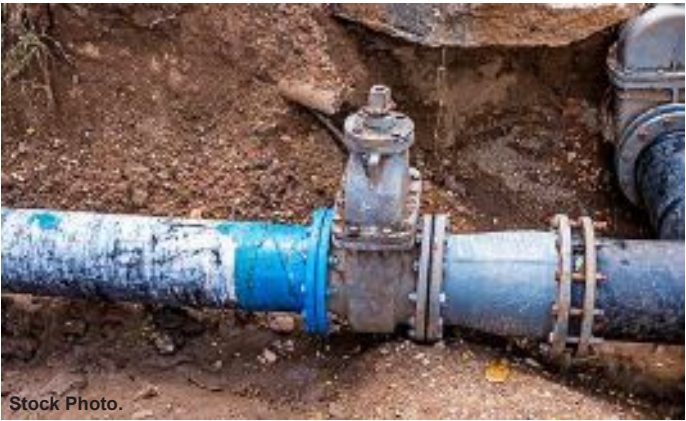
The CRA FY2021 budget proposes funding to assist in the repair of old sewer lines in the CRA to protect the Indian River Lagoon; continue to provide grants for building improvements; and continue to repair and install sidewalks in the CRA.
