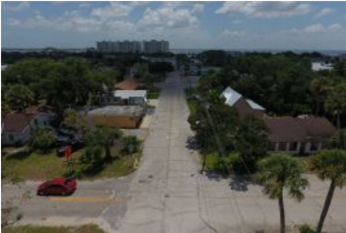
Sidewalk work is scheduled to commence this summer on Lemon Avenue and Broad Street. Also to begin is street resurfacing of Pine Street west of Hopkins Avenue, Orange Street west of Hopkins Avenue, and Lemon Avenue.
