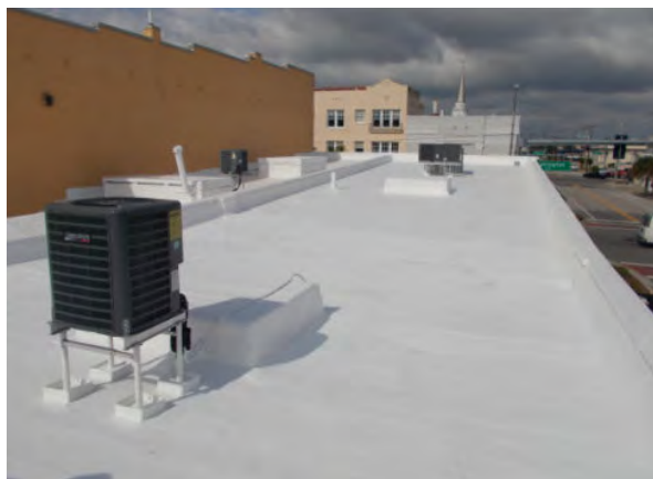
Roof view from the rear of the Museum
